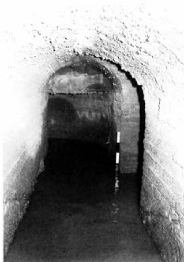
Plate 3.3: Gatehouse subterranean passages; viewed from beneath the front wall, looking west. The photograph shows the high water table that caused problems at the time of construction, 1983 (English Heritage)
