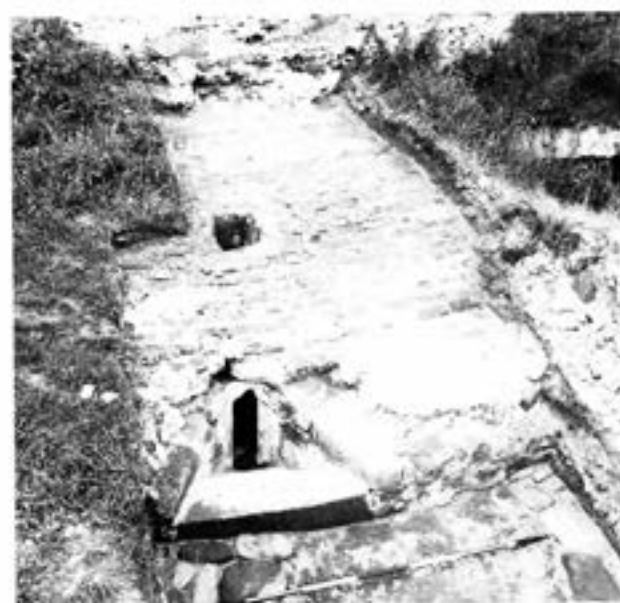
Plate 3.16: The Vaulted Ring Passage; north-west section showing surviving vault from outside, with a gun loop and a smoke vent. 1963 (English Heritage)
