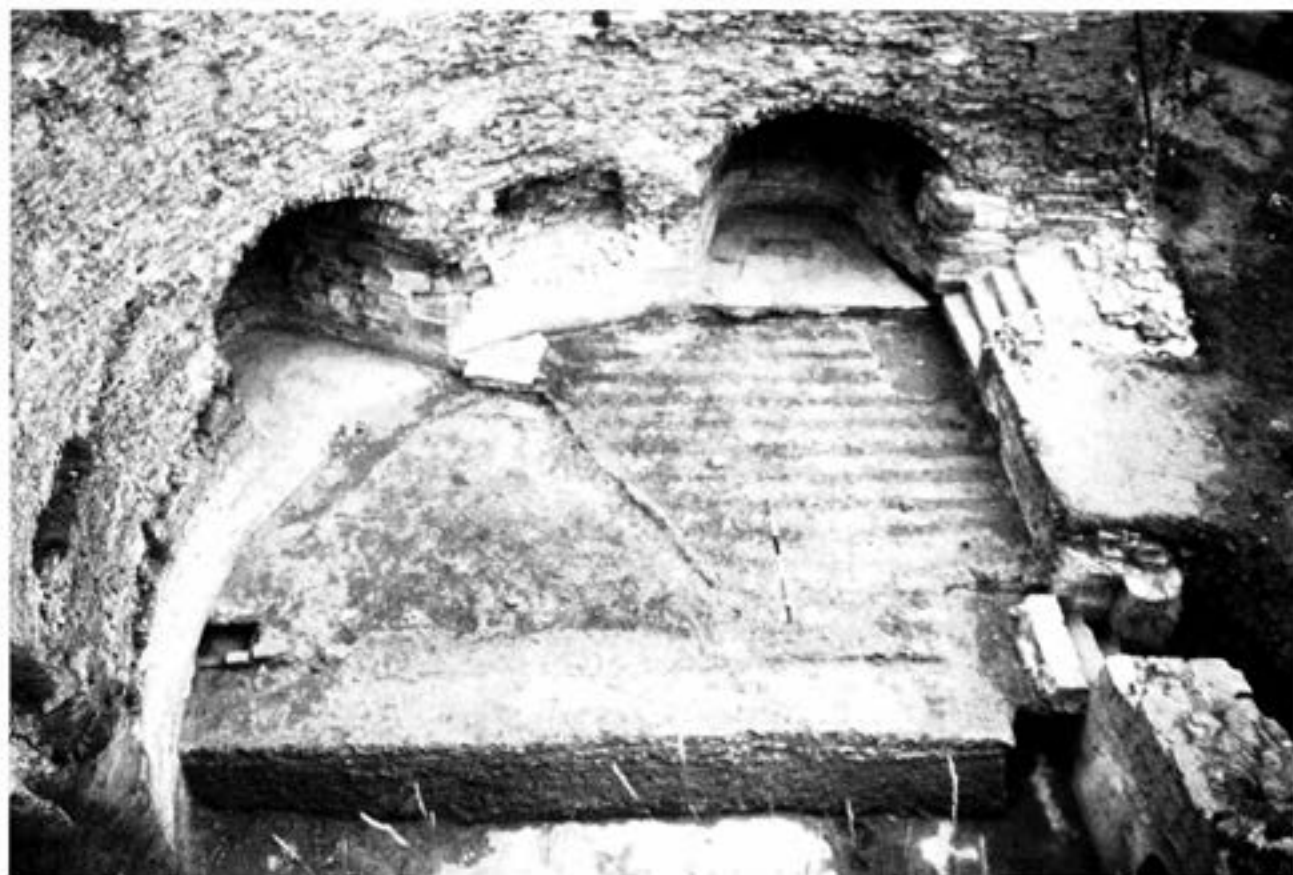
Plate 3.25: W Bastion interior, under excavation in 1973; north and north-west casemates; the displacement of the north casemate to the west bringing it closer to the north-west casemate is clear. (English Heritage/Ames)
