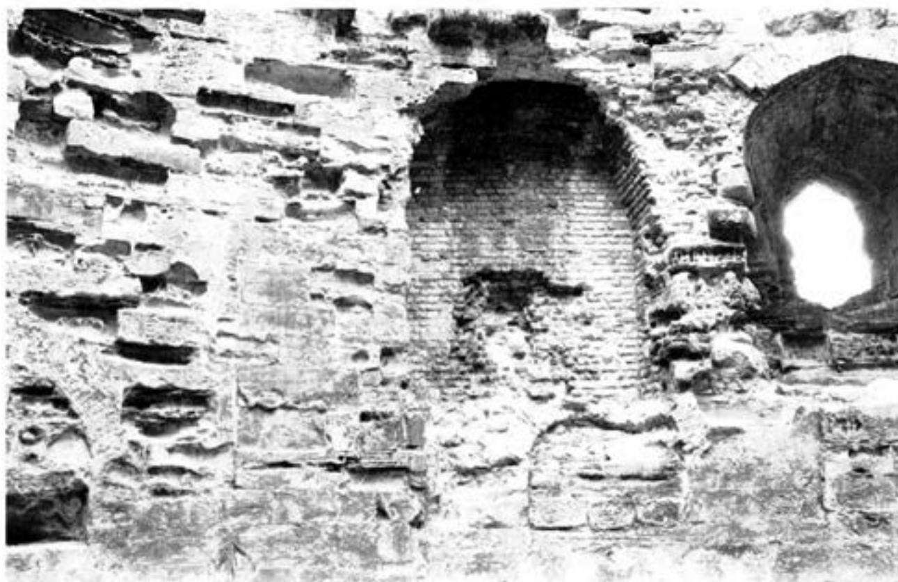
Plate 3.13: The Keep; detail of south-west wall elevation. The replacement fireplace of phase IIb (2115) is visible in the centre of the shot, with the phase IIb west window (2116) immediately adjacent. Below fireplace 2115 is a blocked phase I gunport (2123), and the blocked phase I fireplace (2186) can be seen immediately below the window. The blocked phase Ib door (2185) can be seen on the left of the shot. 1998 (OAU)
