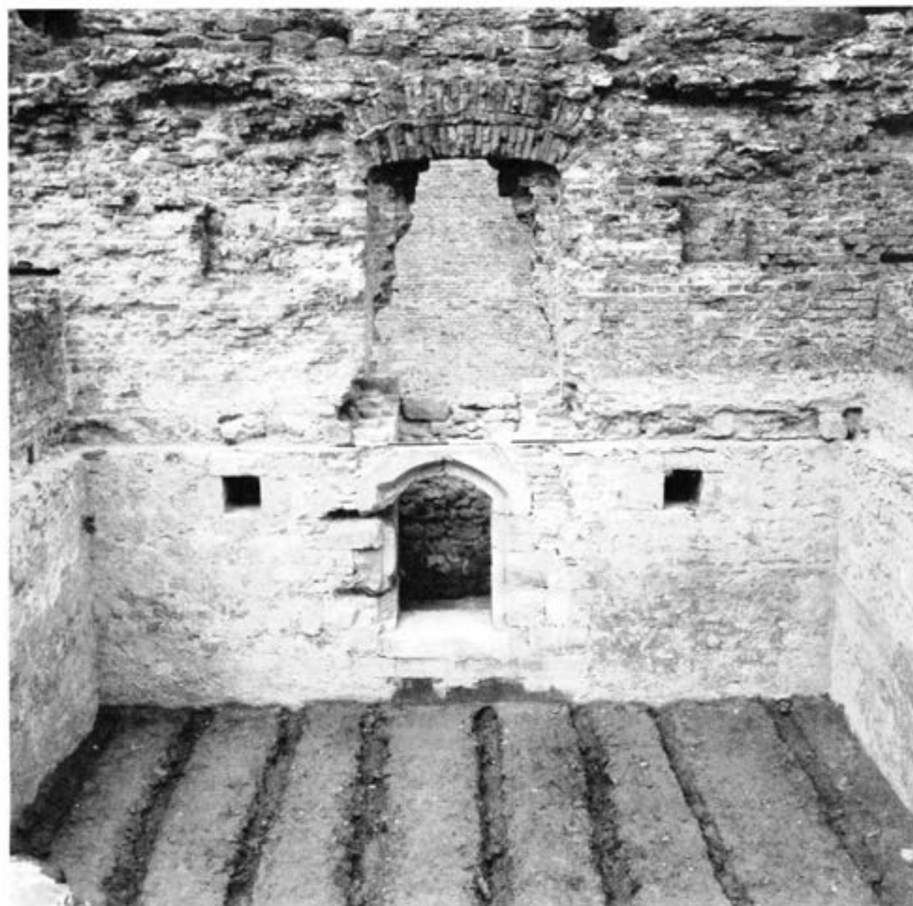
Plate 3.18: The N Stirrup Tower; detail of the chord wall seen from the Stirrup Tower interior, showing openings of phase IIb and phase III, looking north. 1983 (English Heritage/Sheppard)
