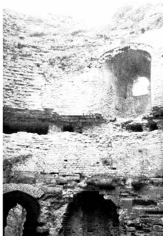
Plate 3.14: The Keep; housing for the phase IIb cannon deck joists. 1963 (English Heritage/Biddle)
