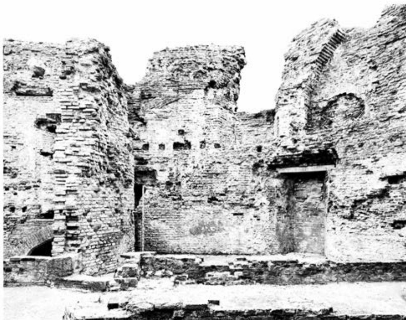
Plate 3.33: Entrance Bastion north-west interior elevation; towards the right of the photograph, at ground floor level, is gunport 2481. Above the gunport are the remains of the brick-arched fireplace 2482, with window 2475 immediately adjacent. The cross-wall dividing the D-shaped bastion from the Gatehouse can be seen towards the left of the photograph; immediately to the right of this wall on the photograph are the remains of joistholes for the floor timbers. 1998 (English Heritage)
