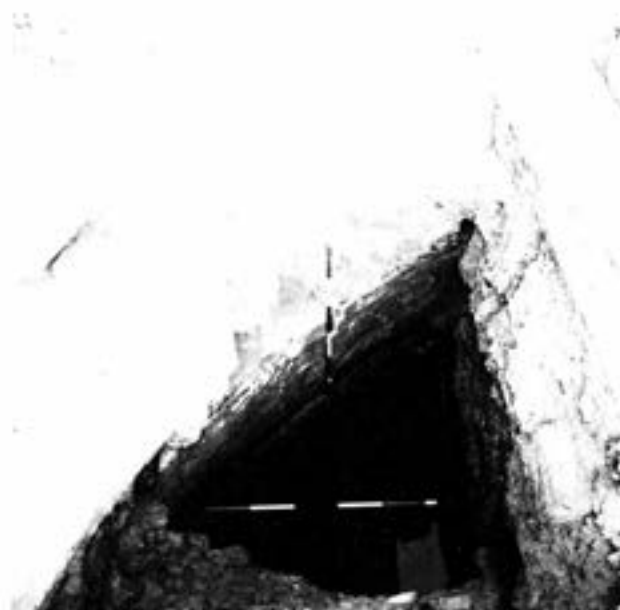
Plate 3.6: The Entrance Bastion N Quadrant Room under excavation in 1965, showing the original sill of gunport 2487 at the abandoned basement level. (English Heritage/Biddle)
