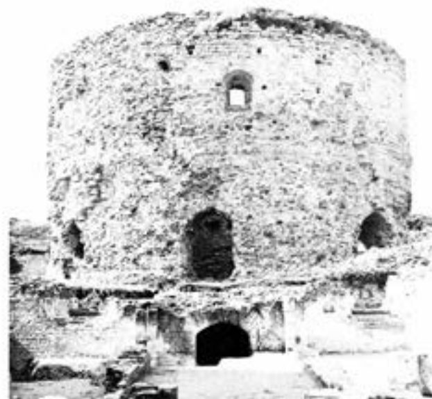
Plate 3.1: The Keep, external view, from the north. The possible phase IIb entrance, aligned with the Entrance Bastion, can be seen in the centre of the Keep wall. In the foreground is the abandoned Vaulted Passage or Cellar, blocked in phase III. 1963 (English Heritage/Biddle)
