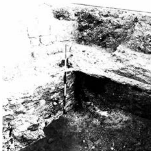
Plate 3.31: Entrance Bastion exterior, looking south; on the right of the picture the phase III ramp to the new Entrance can be seen sloping up above the former outlet of the subterranean passage at the face of the former Gatehouse wall. 1965 (English Heritage/Biddle)
