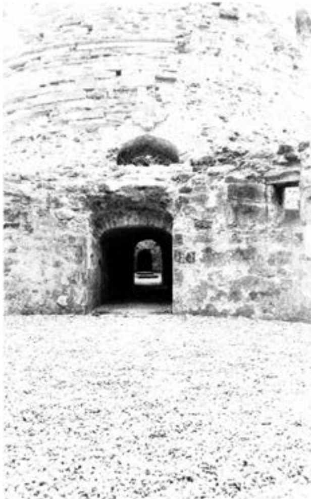
Plate 3.9: The Keep; view from the N Stirrup Tower showing the basement level entrances (north, foreground; south, background) from the Keep into the Vaulted Ring Passage and Radial Passages. Also visible in the surviving wall face are a blocked recess for a decorative plaque, the resited string course, and the two courses of yellow (here shown as light) brick representing the original string course level of the phase I Tower. 1998 (OAU)
