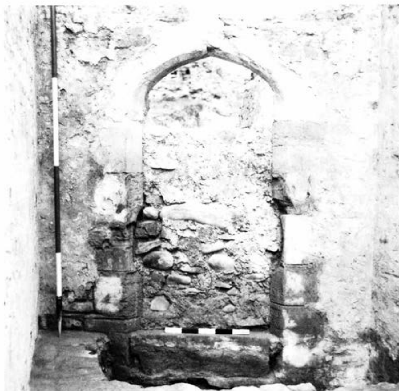
Plate 9.2: WNW Curtain Wall gallery basement, looking north-east to the partially blocked door into the W (Kitchen) Bastion, which may have functioned as a serving hatch. 1982 (English Heritage/Streeten)
