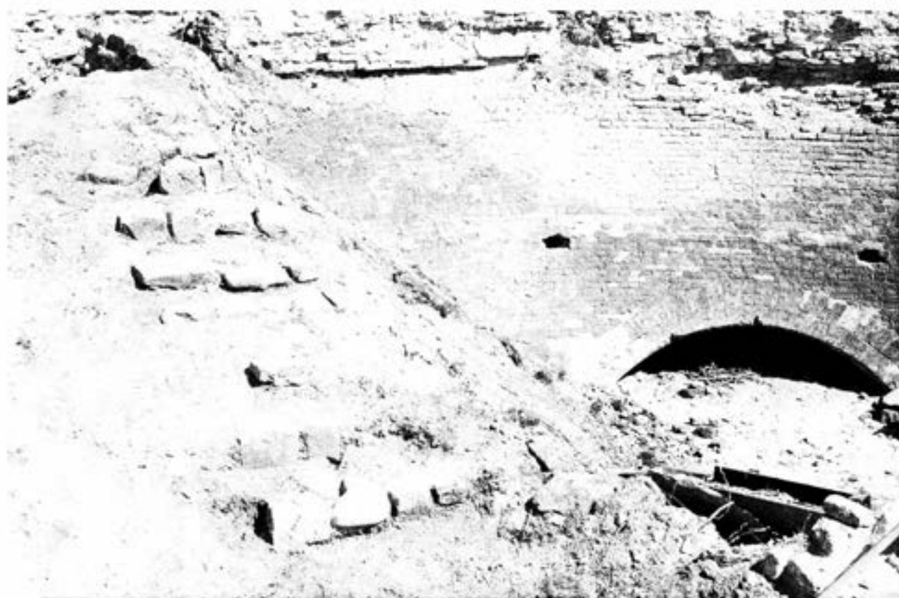
Plate 3.38: The N Bastion, looking north-east; pre-clearance photograph of stone steps set into the top of the bulk fill. 1972 (English Heritage)
