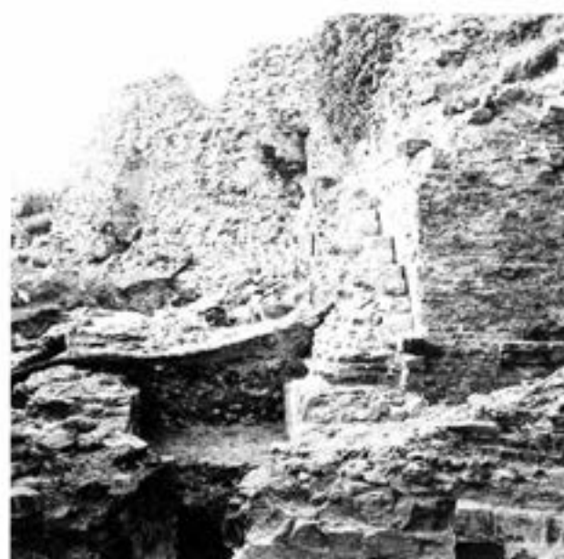
Plate 3.27: E Curtain Wall Gallery looking north; to the right of the picture can be seen the straight joint between the phase IIb and phase III Curtain Walls.
