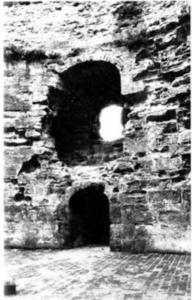
Plate 3.10: The Keep, view from the north showing the south window of phase IIb, above the entrance to the Vaulted Ring Passage. Also visible, above the window, are housings for the phase IIb gundeck joists. 1998 (OAU)
