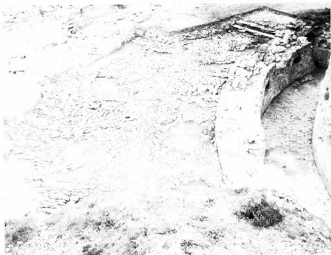
Plate 3.15: The Courtyard and Vaulted Ring Passage; south-western section showing cobbling of courtyard with drain, and the interior of the passage at the point where the original roof structure has gone, looking north. 1983 (English Heritage/Sheppard)
