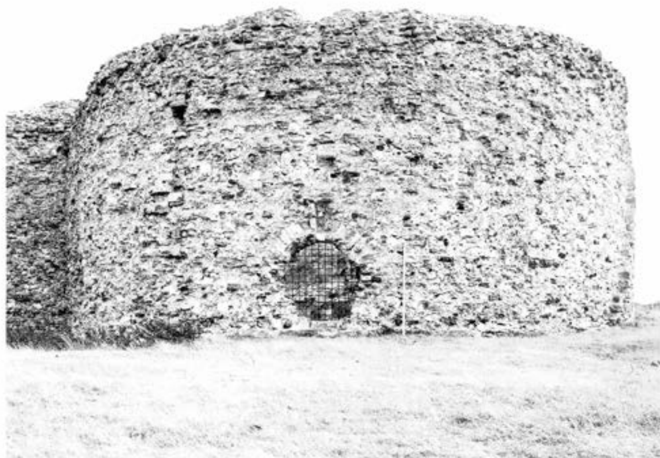
Plate 3.40: W Bastion exterior, looking south-east; showing the enlargement of the NW-facing gunport, perhaps used as a doorway for the removal of salvage material. 1998 (English Heritage)
