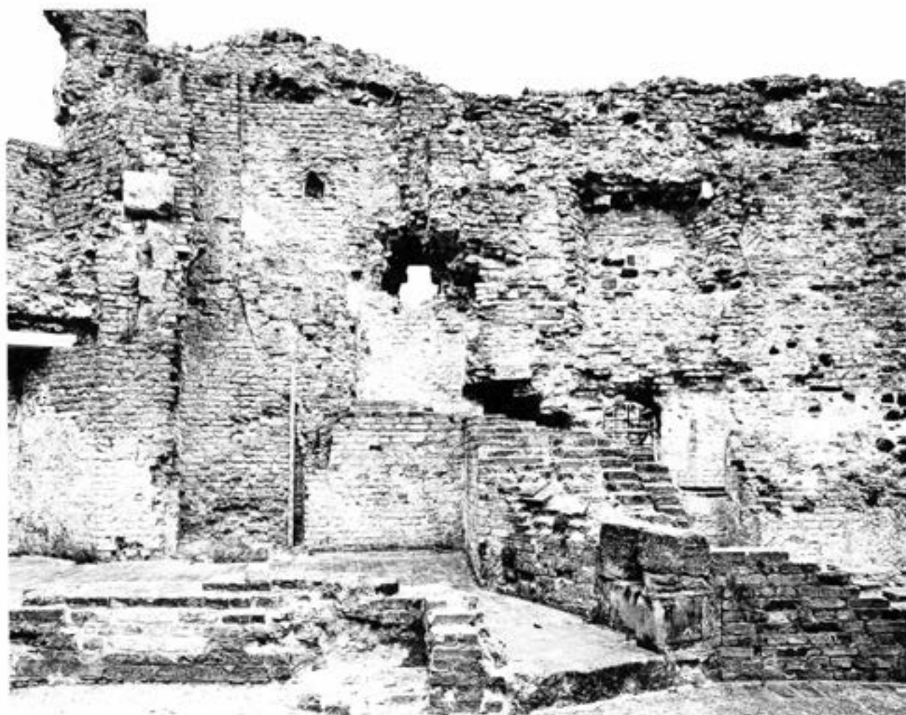
Plate 3.32: Entrance Bastion north-east interior elevation; in the centre of the photograph is the phase III garderobe with external window. To the right of the garderobe is a blocked window; to the left is a chimney with the ground floor fireplace of the N Quadrant Room. On the extreme left is gunport 2487, with window 2486 above. 1998 (English Heritage)
